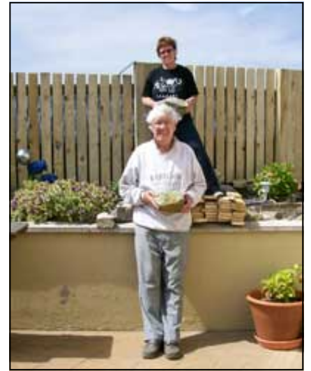
Dad supporting me in my latest venture of building my own fence
